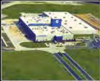
PAGELAND, SC Bronze Foundry and Manufacturing Plant
